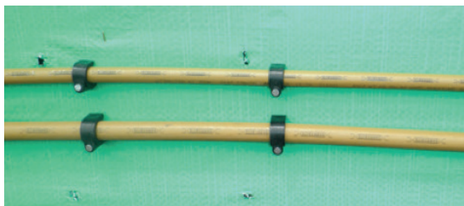
Figure 13.3 Installed piping services prior to the installation of STAAC WALL® panel
